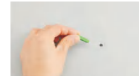
3 Punch holes in each of the two marked positions, insert the expansion screw protective sleeve into the hole of the wall
