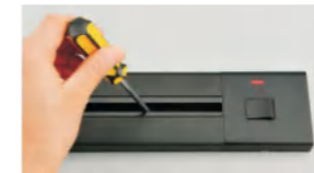
6 Place the track against the wall and screw the track to the wall at the hole position
