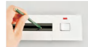
2 After smooth the groove, mark the hole
