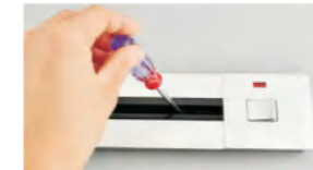
7 Place the track against the wall and screw the track to the wall at the hole position
