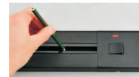
1 Determine the installation location, mark the hole
